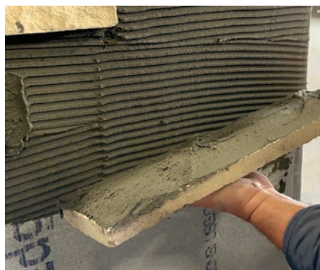
Proper installation with wet-to-wet bond
