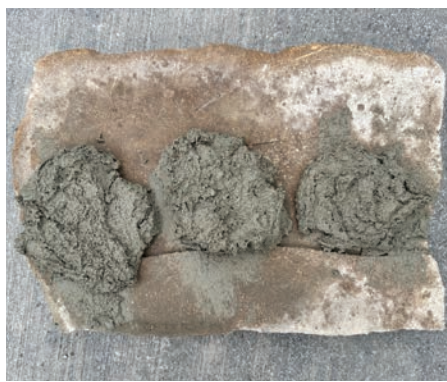
Spot bonding – improper application
