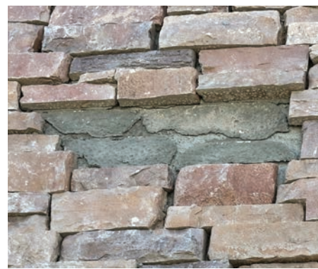
Improper application not 100% coverage leaves air pockets – not wet-to-wet bond
